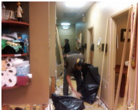
Workers from a cleaning crew tear up carpets, baseboards, drywall and anything else that got soaked in Dr. Snyder's Ship Bottom, N.J., office.
